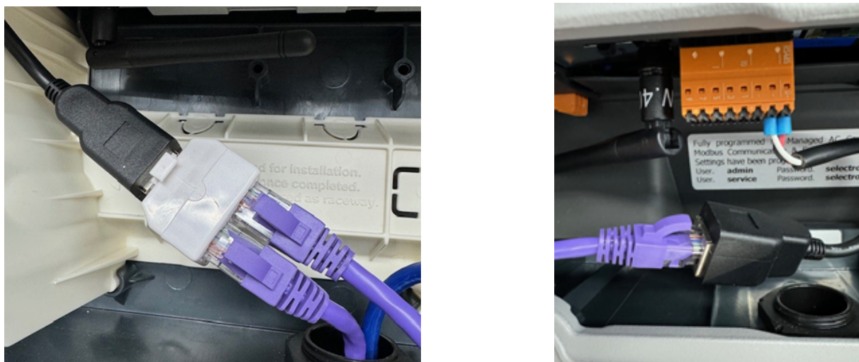
Fig 9: Ethernet cable to AC Coupled inverters (Left: Gen24 Right: SnapINverter)
