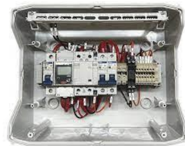
3 rd party backup boxes
